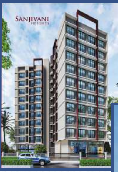
SANJIVANI HEIGHTS DAHISAR (EAST) (COMPLETED)
